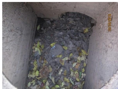
Catch Basin at street level and inside with debris before cleaning
