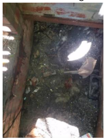
Catch Basin after cleaning
