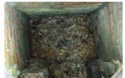
Catch Basins with grates holding water and debris
