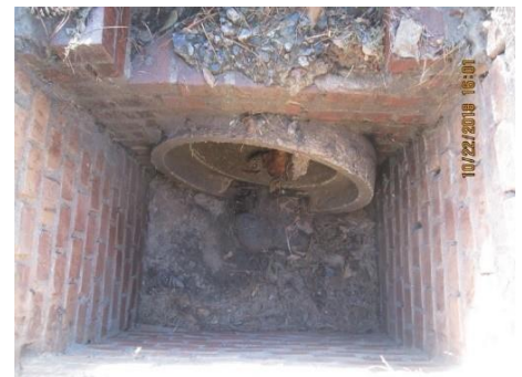
Catch basin after cleaning
