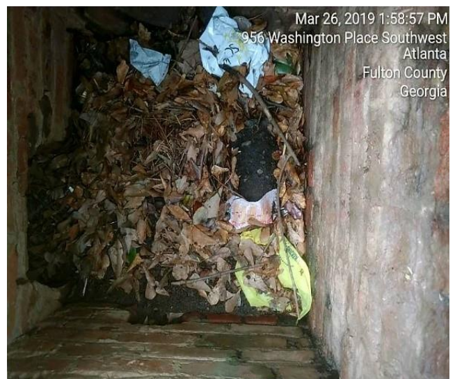
Catch Basins severely compromised with leaves, trash and debris
