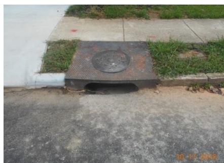
Debris outside and inside Catch Basin
