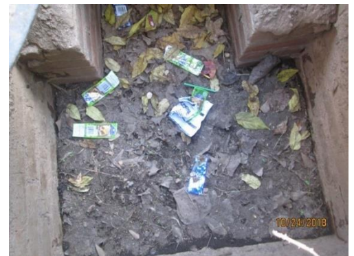
Interior of Catch Basin
