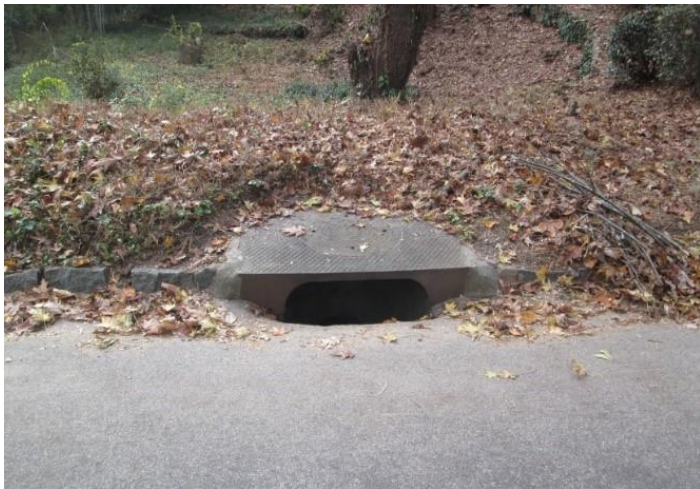
Catch basin with heavy debris inside and at inlet
