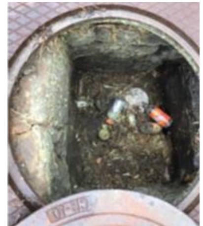
Catch Basin before
