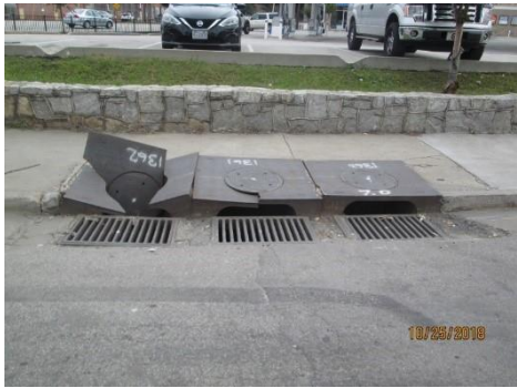
Triple grated inlet damage and in need of cleaning
