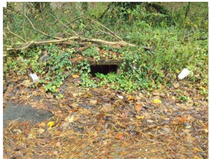
Two catch basins severely compromised with debris and overgrowth
