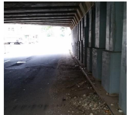
Underpass Catch Basins
