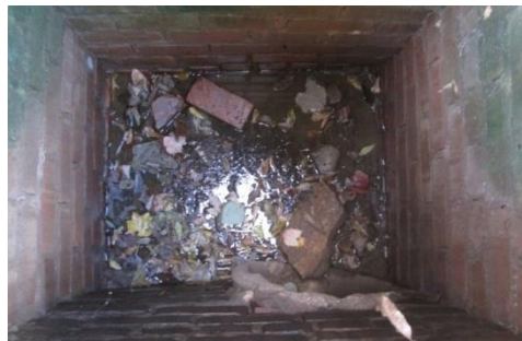
Heavy debris inside and out at Catch Basin
