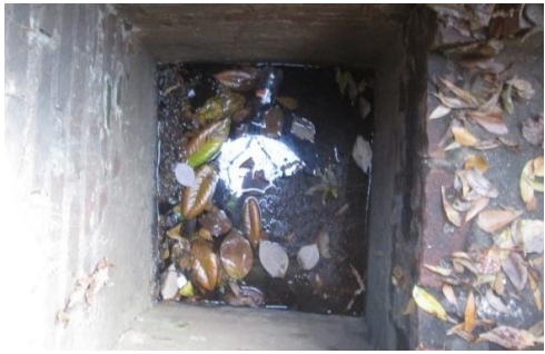
Catch Basin with heavy debris and holding water
