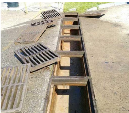
Multi-grate system before and after cleaning
