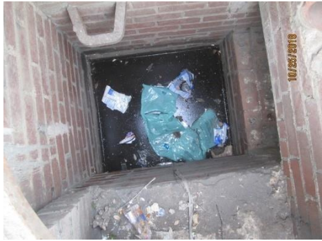
Triple grated inlet damage and in need of cleaning
