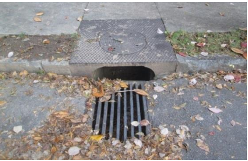
Catch Basin with heavy debris and holding water
