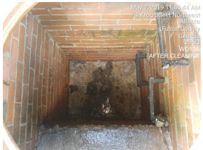
Catch Basin after cleaning
