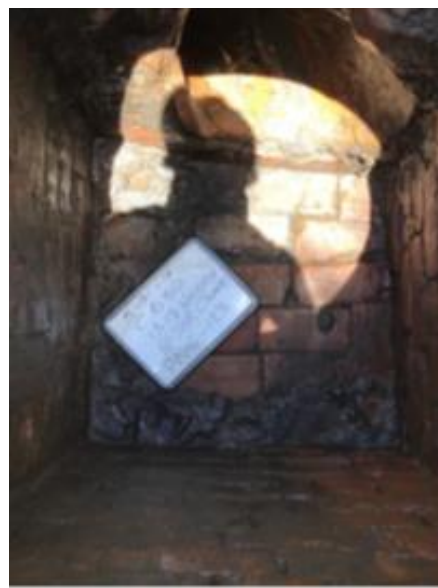
Catch Basin severely compacted with debris before
