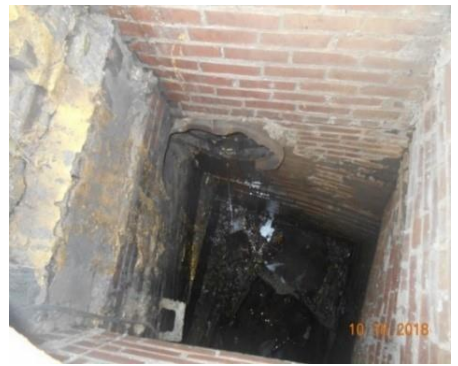
Triple gate ready for cleaning
