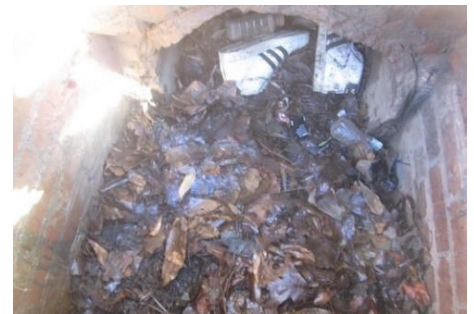
Comprised Catch Basin before cleaning
