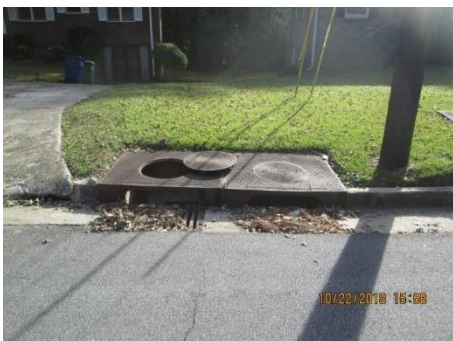
Double Catch Basin with grates full of leaves
