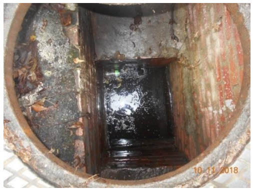
Catch Basin holding water before cleaning
