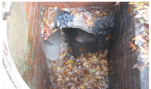
Heavy Debris in Structure
