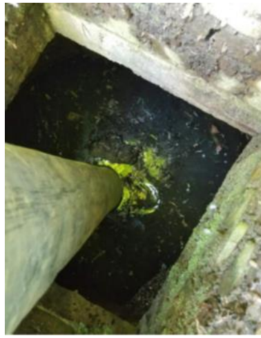
Vector cleaning of Catch Basin and results
