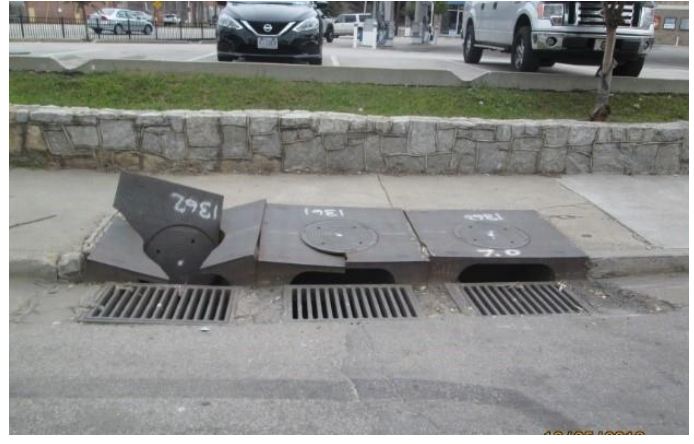
Street view and broken Catch Basin tops
