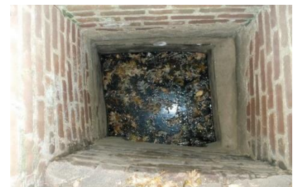
Catch Basins with grates holding water and debris
