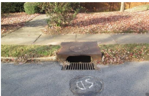
Debris at curb-line and within Catch basin
