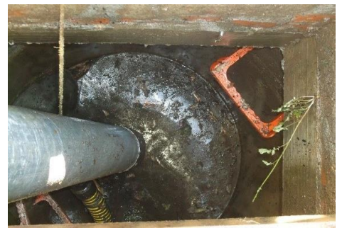
Vactor Truck Cleaning a grated drain
