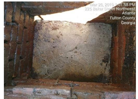
Drop Inlet after cleaning
