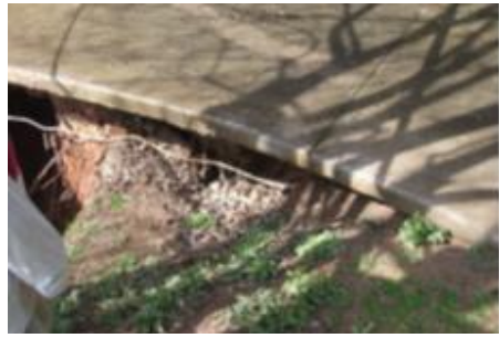
Sidewalk failure, sink hole on private property
