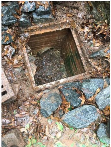
Drop Inlet after cleaning
