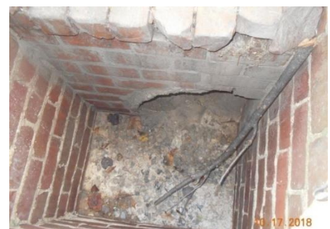
Debris outside and inside Catch Basin
