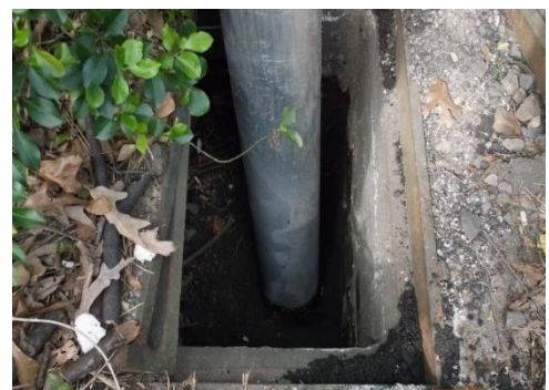
After Cleaning; ready for CCTV
