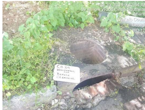
Catch Basin before cleaning-plastic bottles, cans, other debris
