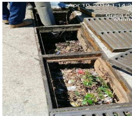
Multi-grate system before and after cleaning
