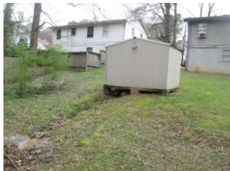
Private storage unit on top of headwall
