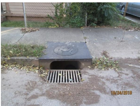
Catch Basin at street level and inside with debris before cleaning
