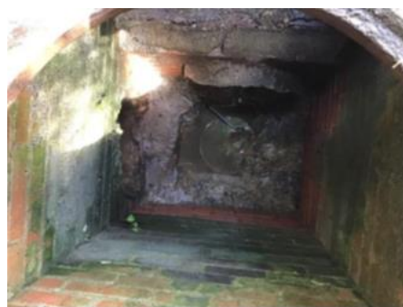
Vactor cleaning Catch Basin
