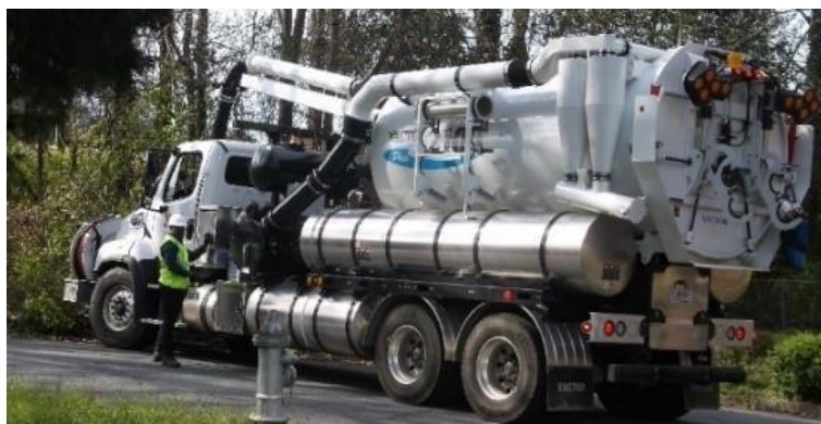
VAC Cleaning Grate Inlet
