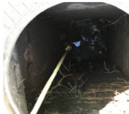
Catch Basin after cleaning
