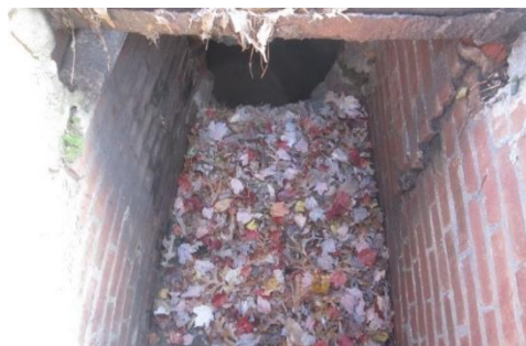
Debris at curb-line and within Catch basin
