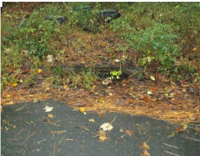
Two catch basins severely compromised with debris and overgrowth
