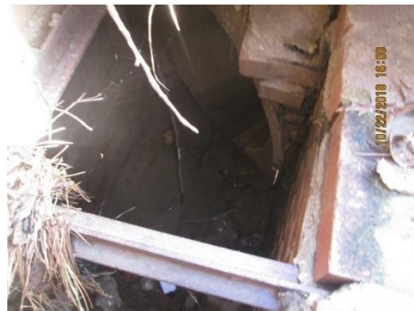
Roots and grass clippings before cleaning
