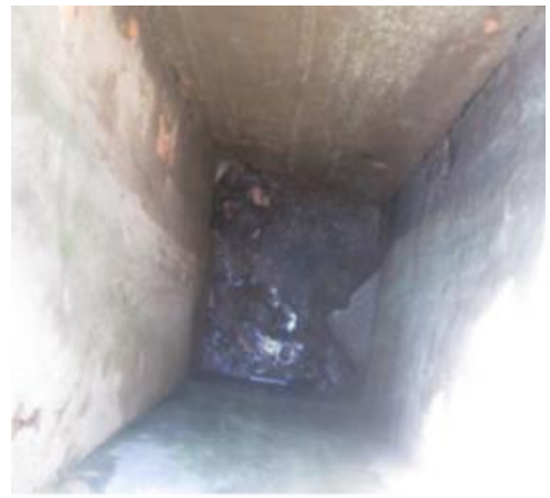
Catch Basin after cleaning
