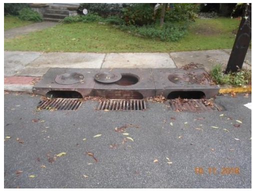
Catch Basin holding water before cleaning
