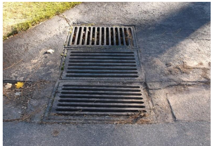
Triple grate in driveway before cleaning
