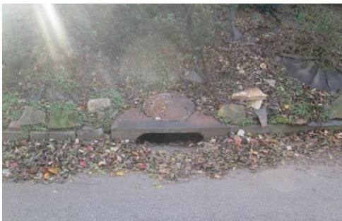
Heavy debris inside and out at Catch Basin
