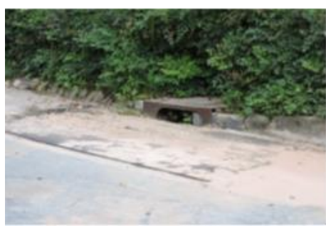
Catch Basin at roadway
