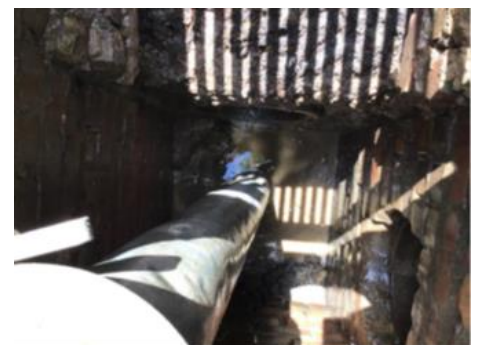
Cleaned Catch Basin
