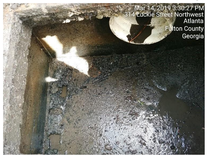
Drop Inlet after cleaning
