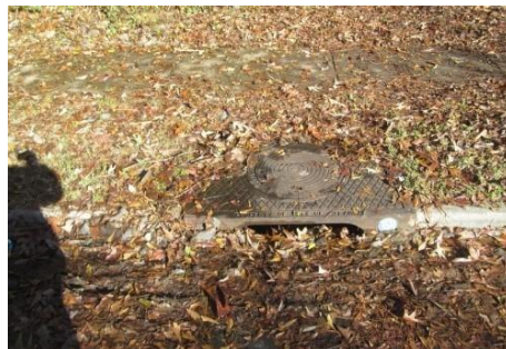
Comprised Catch Basin before cleaning
