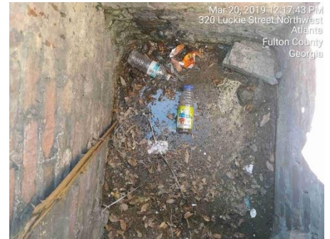
Drop Inlet before cleaning
