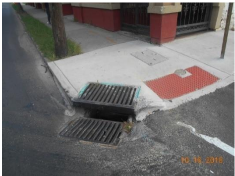
Grate Inlet at Surface
