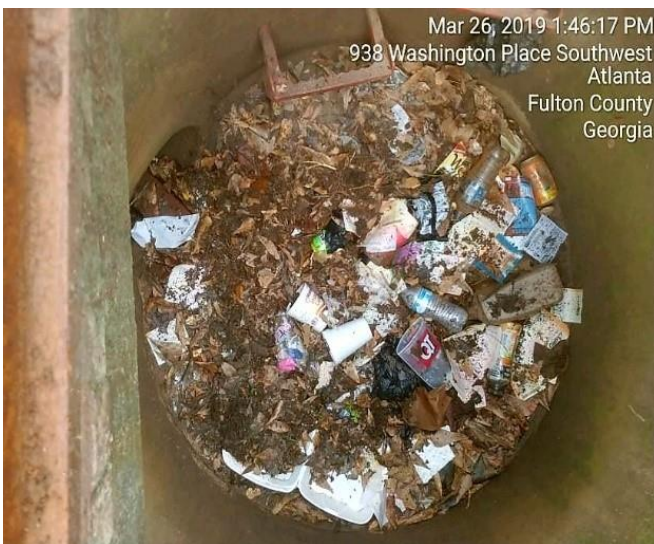
Catch Basins severely compromised with leaves, trash and debris
