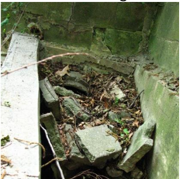
Collapsed headwall
