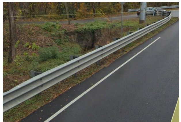
Ditch and culvert looking south
