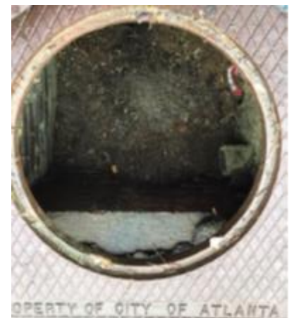
Catch Basin after cleaning
